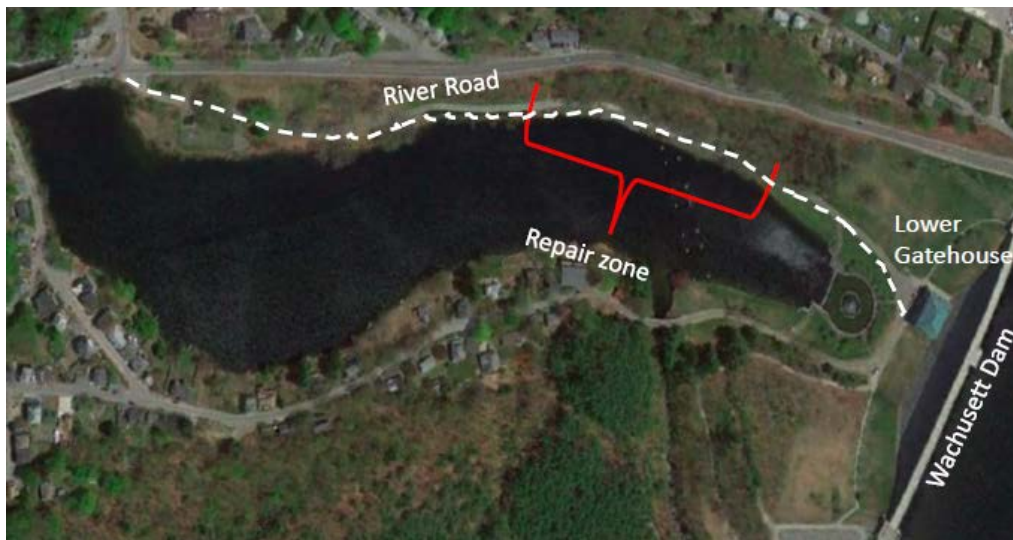
Figure 2. River Road at Wachusett Dam and Lower Gate House
