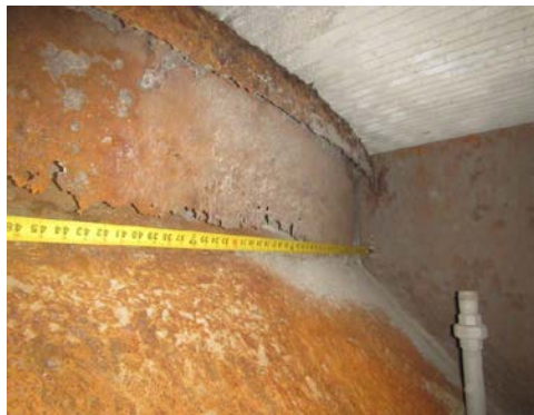
Perforated Closure Plate at Dome/Shell Interface, Right Side
