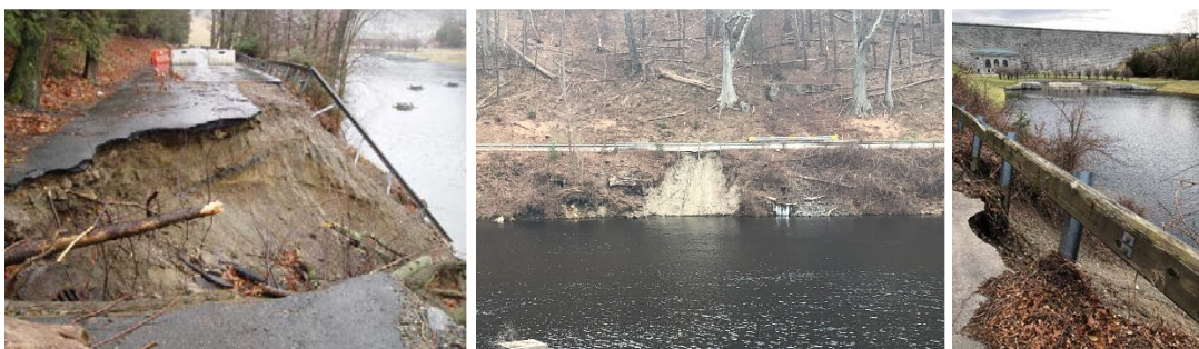
Figure 1. River Road 2008 landslide (L) and 2019 landslide (C) and (R)
