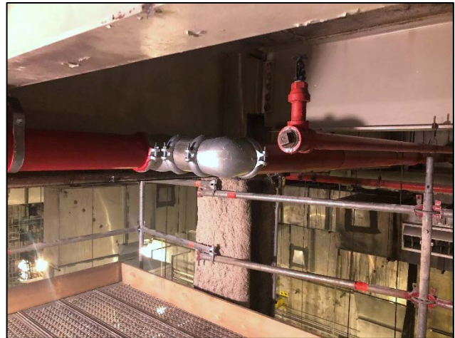
Sprinklers Cut and Capped and Rerouted
